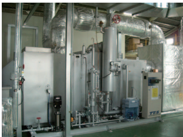
Fig. 3 Heat recovery steam generator
